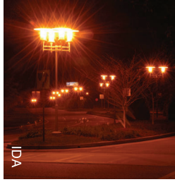
Glaring lights can distress the eyes. The brightest, most visible objects in the area are the lighting fixtures, not the roadways, walkways or parking areas Atlanta, Georgia.
